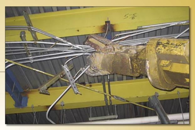
design allowed them to provide a small tool that could be mounted on a mini-excavator. Additionally, they could offer a third member configuration that would afford Watral the ability to reach, rotate, remove and process targeted materials easily. This configuration would also allow him to virtually eliminate the use of man-lifts and substantially increase productivity.
