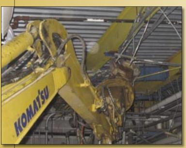
due to limited access, they faced a major challenge in terms of material handling. Everything they removed would need to be sized to fit into a skid steer bucket so it could be transported out of the basement level. This required all materials to not only be removed, but to also be processed within the confined basement area. Additionally, the building's structural sup-
