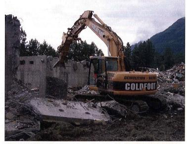
20 was instrumental in completing both projects well ahead of schedule. According to Rodriguez, the MT Shear Jaw Set brought down the fish processing facility with a month to spare, saving the company hundreds of man hours that would have been spent torch-cutting the heavy steel structure.
