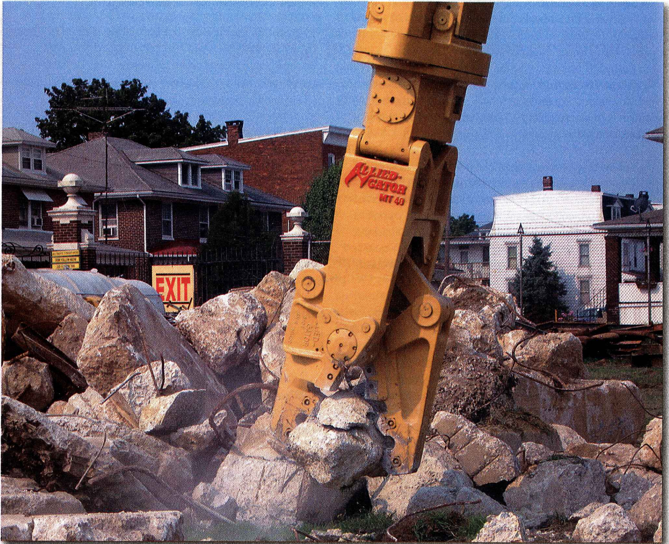
▲ The jaws of an Allied-Gator multi-tool cut through concrete debris and rebar in a snap. Photo by Brian Richesson
