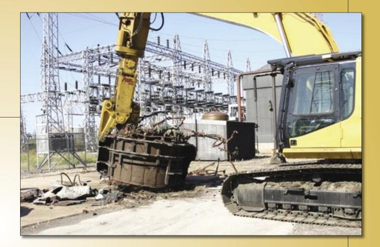
but also two very clean material streams. "It only took me a half hour to break up the whole generator and pull out the copper," says Keith. Looking back on the project Gordon says, "Without that tool, this project would not have been nearly as successful."
