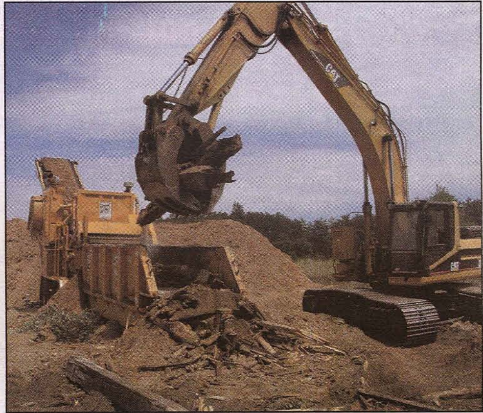
A Bandit 3680 horizontal grinder was used to process pallets and cribbage.
