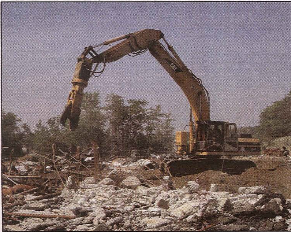
"Pitsch Enterprises interchanges the Allied-Gator MTR 40 S (pictured) with the Allied-Gator ME 40 Mag Extension which increases versatility by giving them the ability to shear and mag with one machine."
