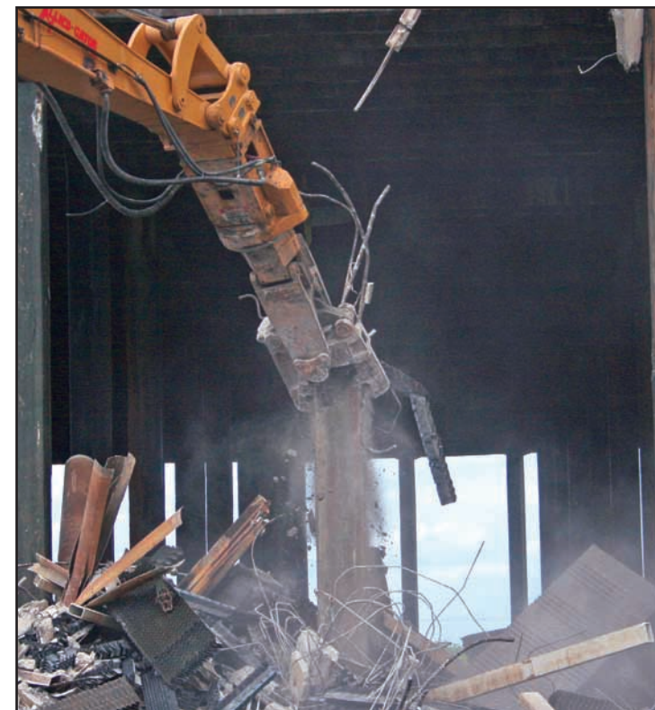
Allied-Gator's MTR 40 Multi-Tool in action.
