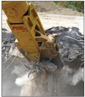
B.O.G. demolishes thick concrete on the Cadiz bridge with the MTR 50 C.
