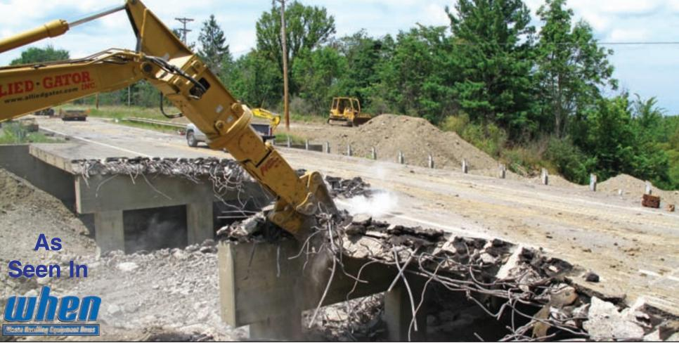
The MTR 50 C cleanly removes rebar from the concrete and leaves perfect fill material.
